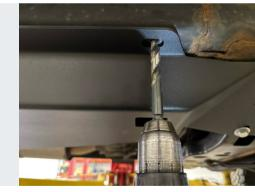
Using the shout as a guide, Mark the center and drill it to accept a 1/2" bolt
