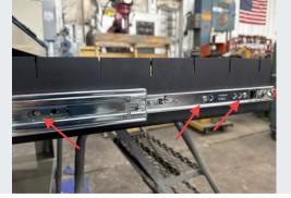
With the to pair of slides fully extended, install top drawer onto the slides using 3x #10 x 1/2" button head screws and flange nuts per side. Ensure that the screws run from the outside in.
