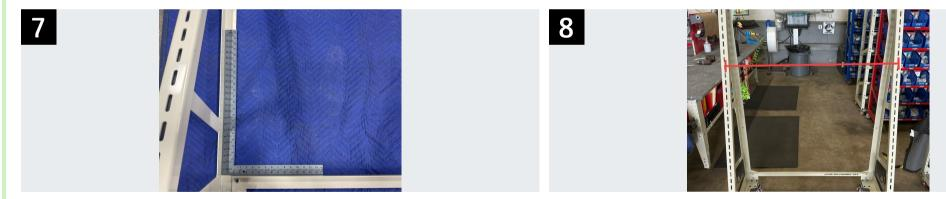
Using a framing square at multiple points, verify that the assembly is square. Once verified, tighten all of the fasteners.
